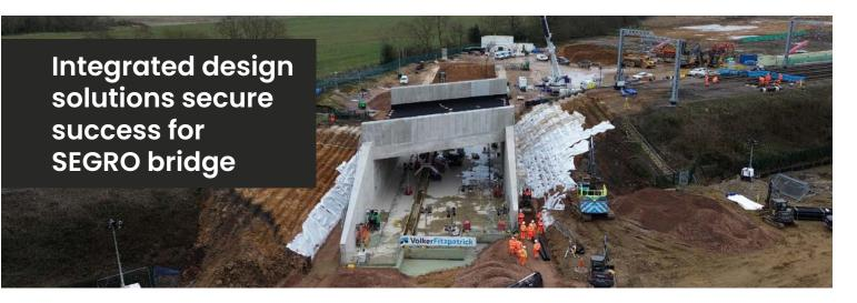
A new reinforced concrete box intersection bridge has been successfully installed under the four-track Midland Main Line between Radlett and St Albans.
