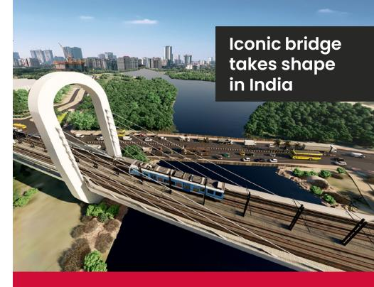
Tony Gee is involved in a new project to build the Shunya Bridge in Mumbai, India. This is a cable stayed bridge set over the Vakola Nala branch of the Mithi River. It is an iconic structure supporting a 130m stretch of the Mumbai Metro and was developed by Indian architectural firm Designfakt with Tony Gee as the lead designer.
