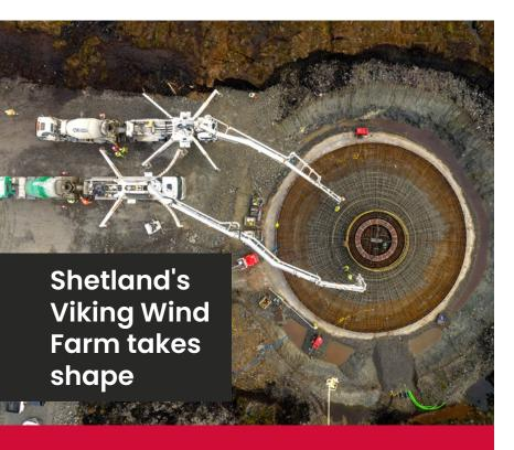
The pouring of concrete on the final wind turbine base marked a major milestone at the Viking Energy Wind Farm on Shetland.
